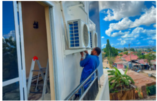
Installing an outdoor unit on a house
