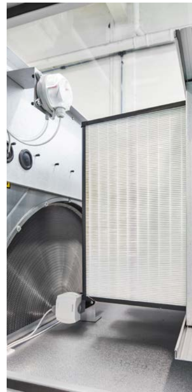
Heat recovery wheel and filter
