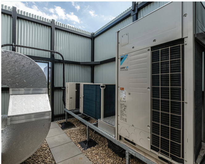
VRV 5 Heat recovery unit recovering waste heat from cooling areas for other heating
