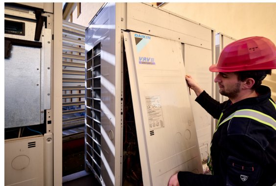
Electrical work formed part of the system's testing and commissioning phase.
