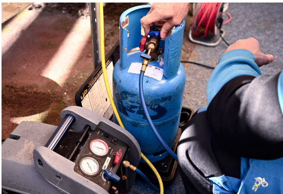
Pumping out the refrigerant into special containers for recovery and subsequent handling in accordance with applicable regulations.
