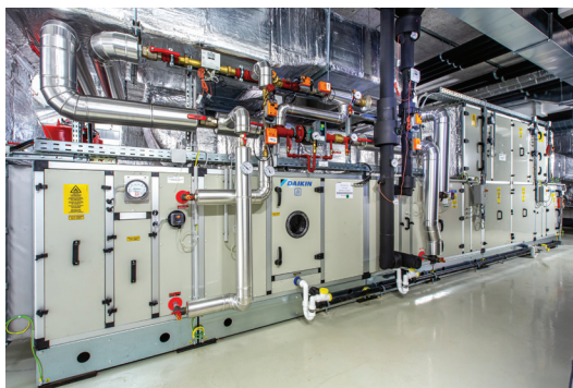
The Daikin Professional Air Handling Units, installed in the basement and on the roof, are all "A" certified according to ErP regulations
