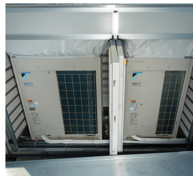
VRV units providing heating and cooling for Your Daikin World
