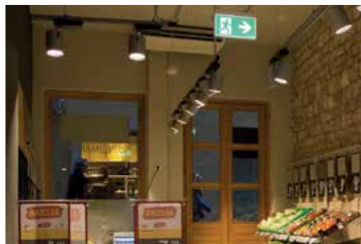
The quiet and discrete indoor units were ideal for the sensitive historic building.
