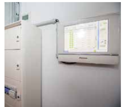
Daikin's intelligent Touch Manager controls the entire HVAC system and is linked with the mall's Building Management System.
