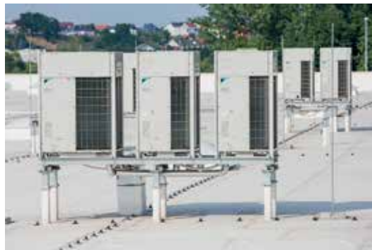
VRV IV monovalent systems heat eight non-food units in the retail park.
