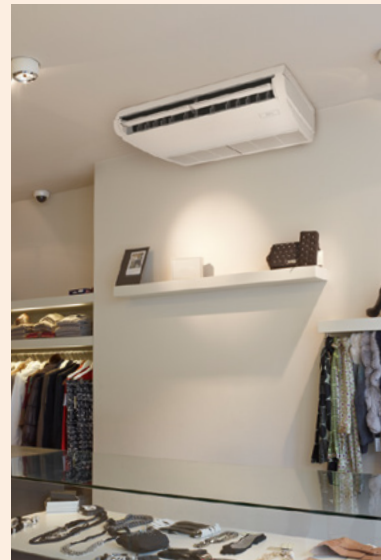
Ceiling suspended unit
