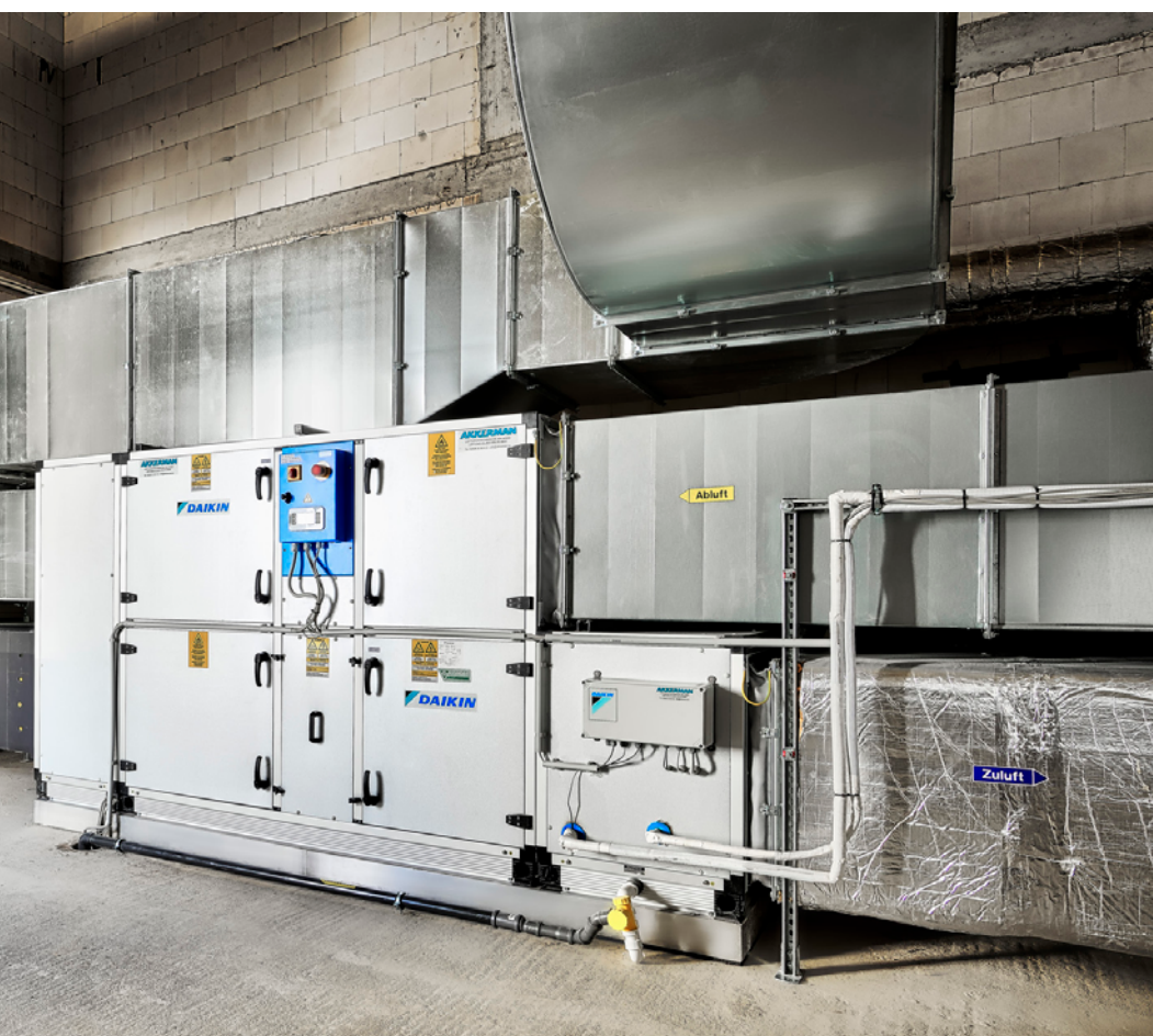
D-AHU Modular R installation
